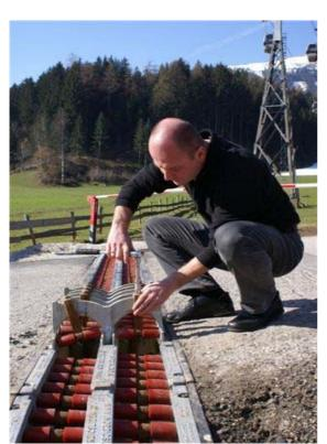
3) Fix the roller elements in horizontal position. Max. torque 25 Nm.
