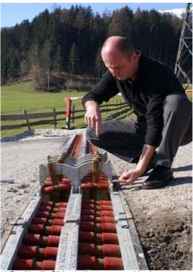
Put Nordic Slider in the gutter upside down.
